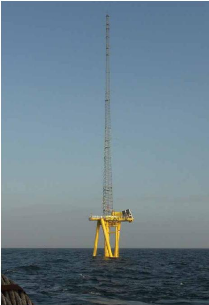
Figure 14 – Completed met mast with helical jacket foundation (October 2011).
